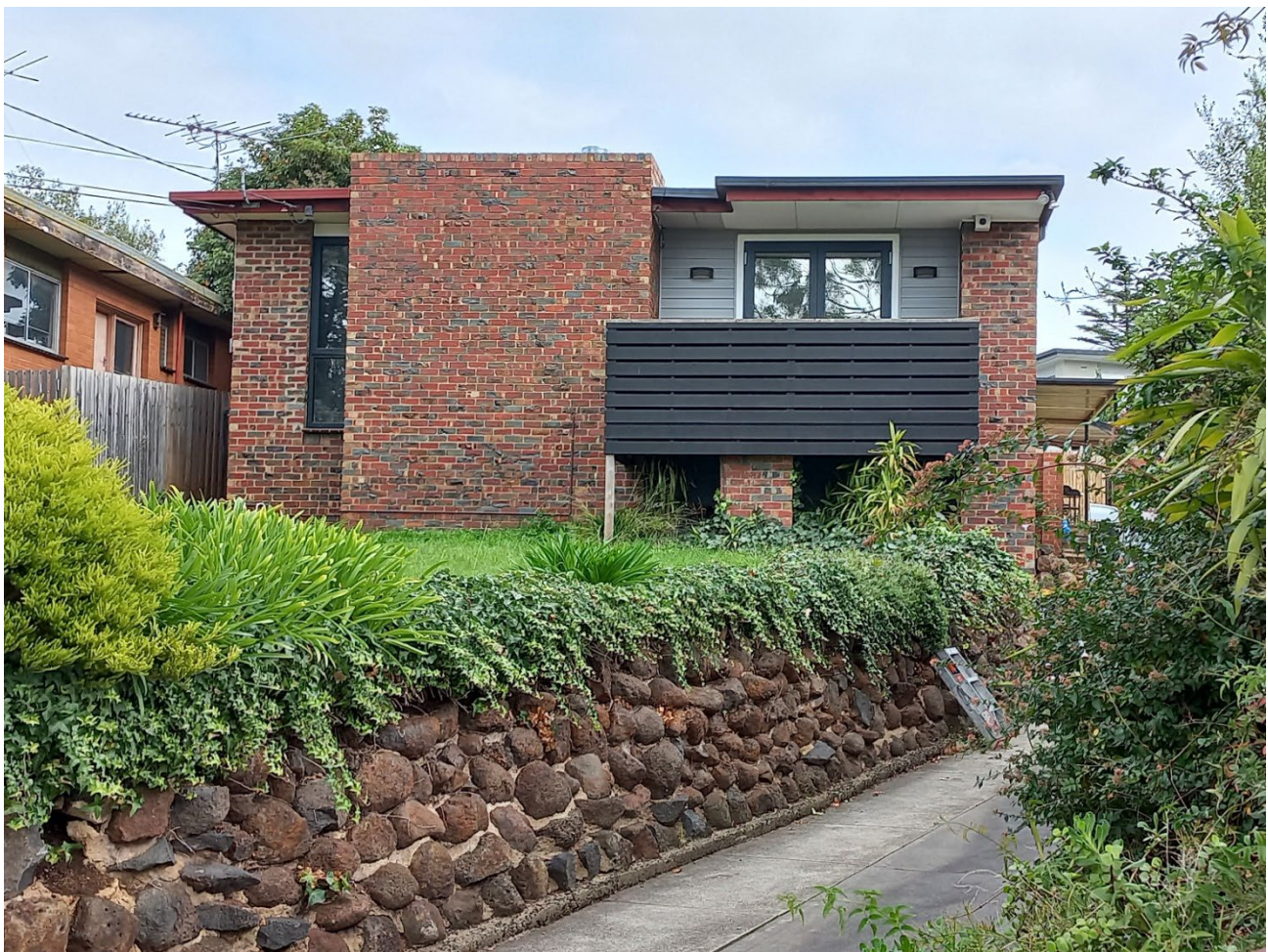
43 Woolart Street, Strathmore. Photographs by Built Heritage Pty Ltd, May 2022
