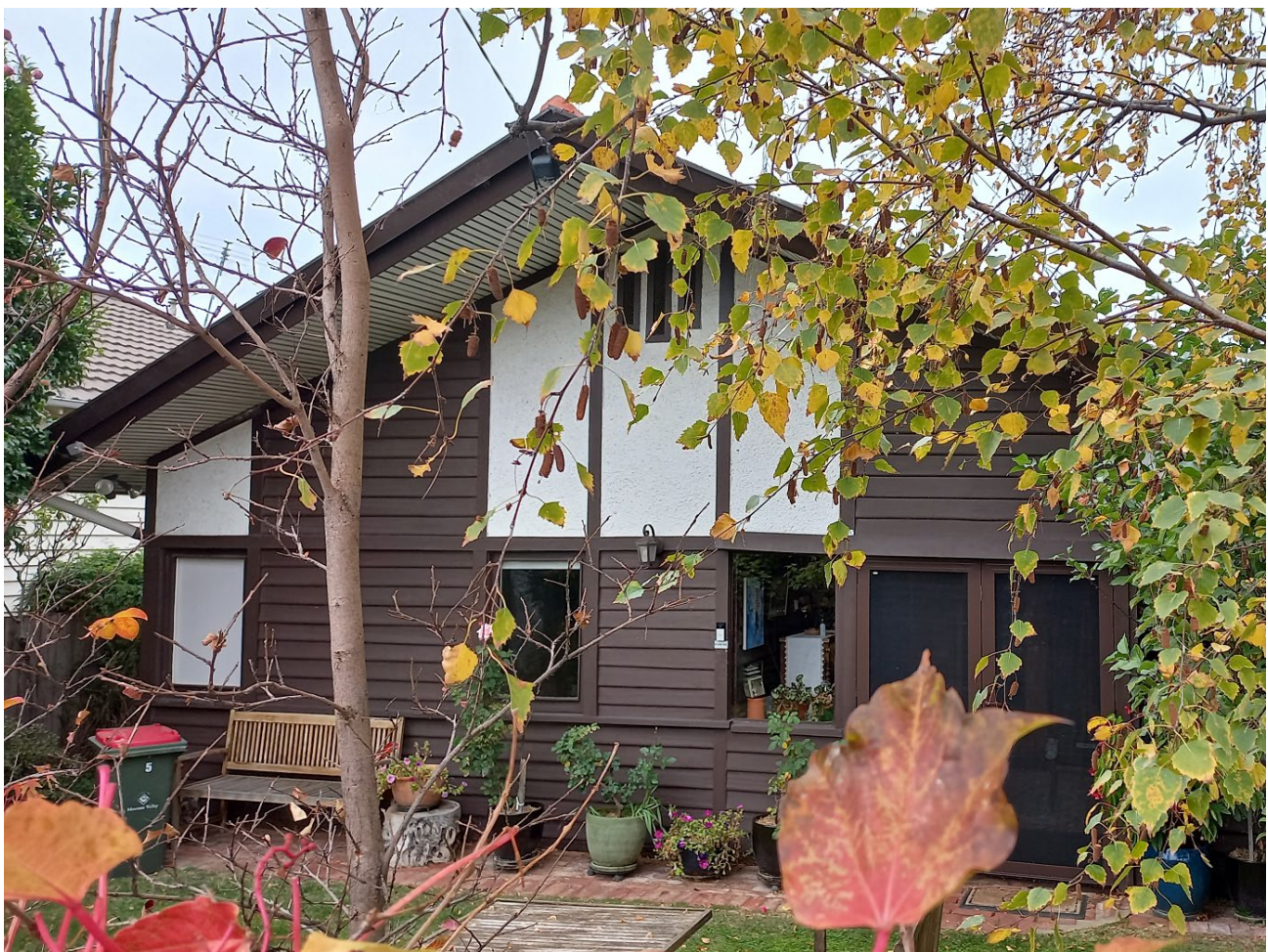
5 Ophir Street, Moonee Ponds. Photograph by Built Heritage Pty Ltd, May 2022
