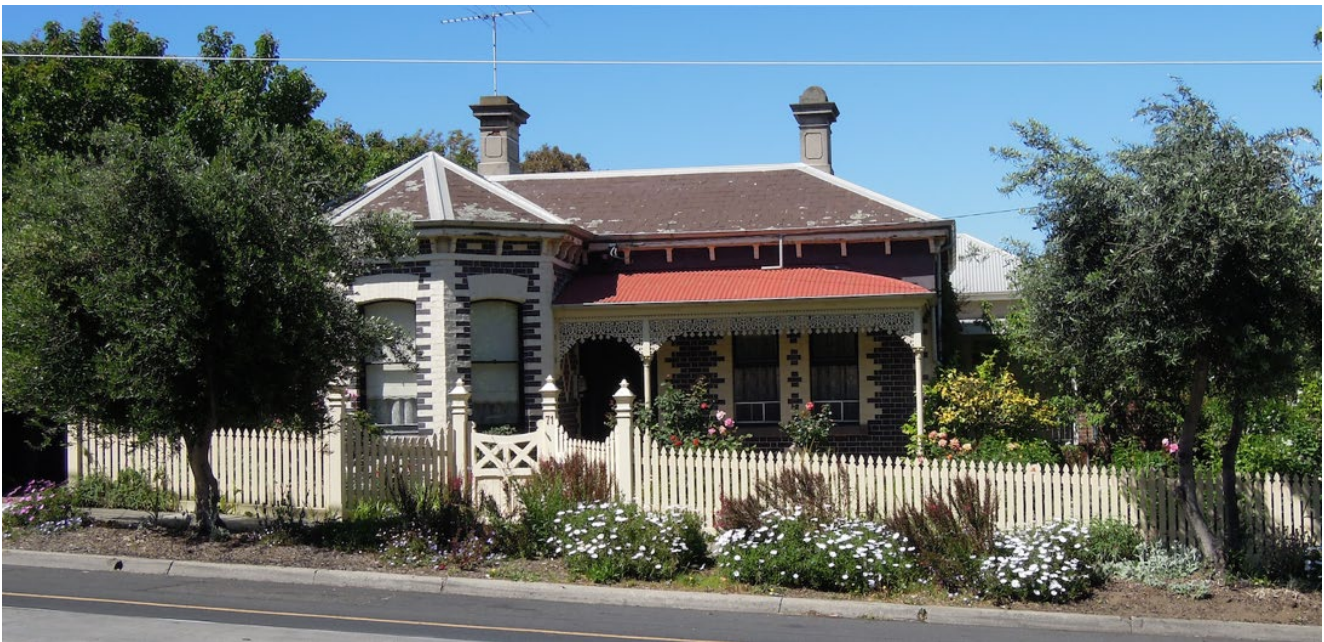
71 Maribyrnong Road, Ascot Vale. Source, M. McDougall, June 2021
