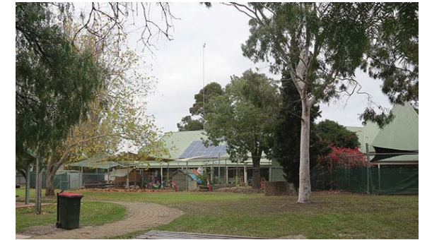
Montgomery Park - existing children's centre building
