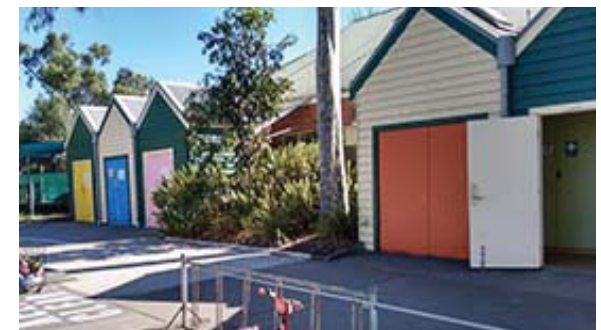
Montgomery Park - Essendon Traffic School - existing toilets and storage structures
