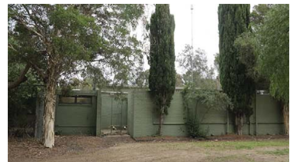
Montgomery Park - disused public toilets at rear of existing kindergarten building
