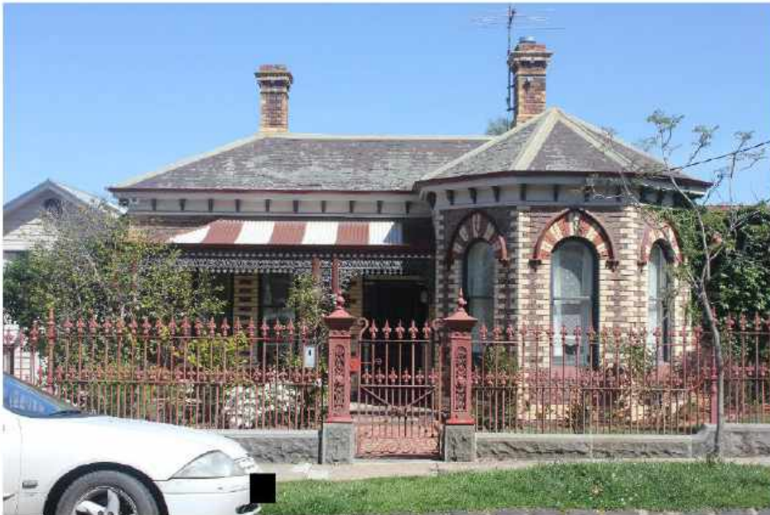
Figure 30. 32 Robb Street, Essendon, principal elevation (source: Context 2018)
