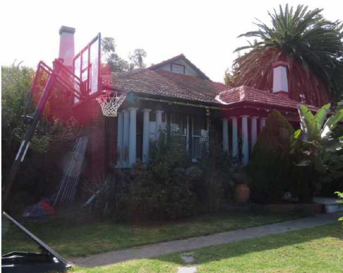
Figure 1. 2 Aberdeen Crescent, Essendon, principal elevation (source: Context 2018)
