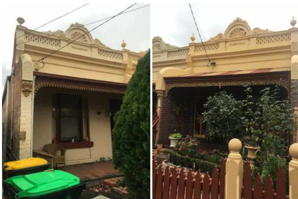
Figures 1 & 2. 21 and 23 Nicholson Street, Essendon, principal elevation (April 2018) (source: Context, 2018)
