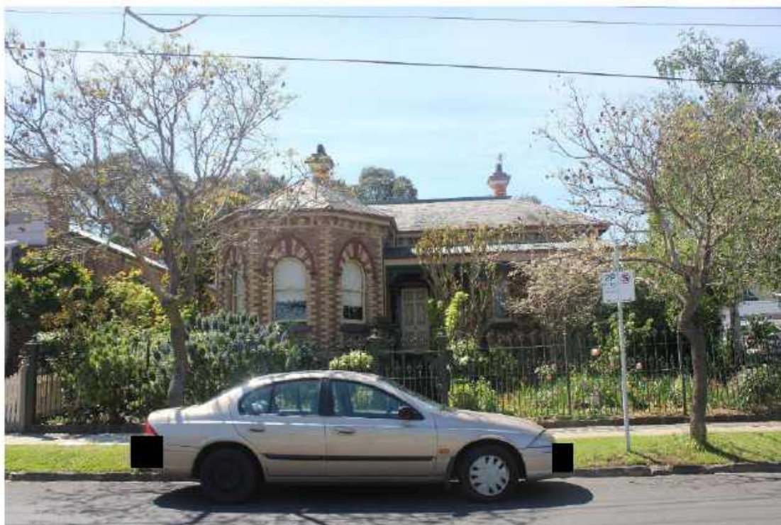
Figure 29. 27 Robb Street, Essendon, principal elevation (source: Context 2018)
