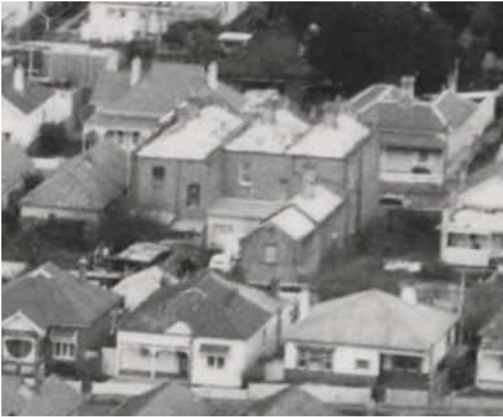
Figure 36 Extract from Charles Daniel Pratt aerial photograph showing 14 and 16 Spencer Street, c1950-60 (source: State Library Victoria)
