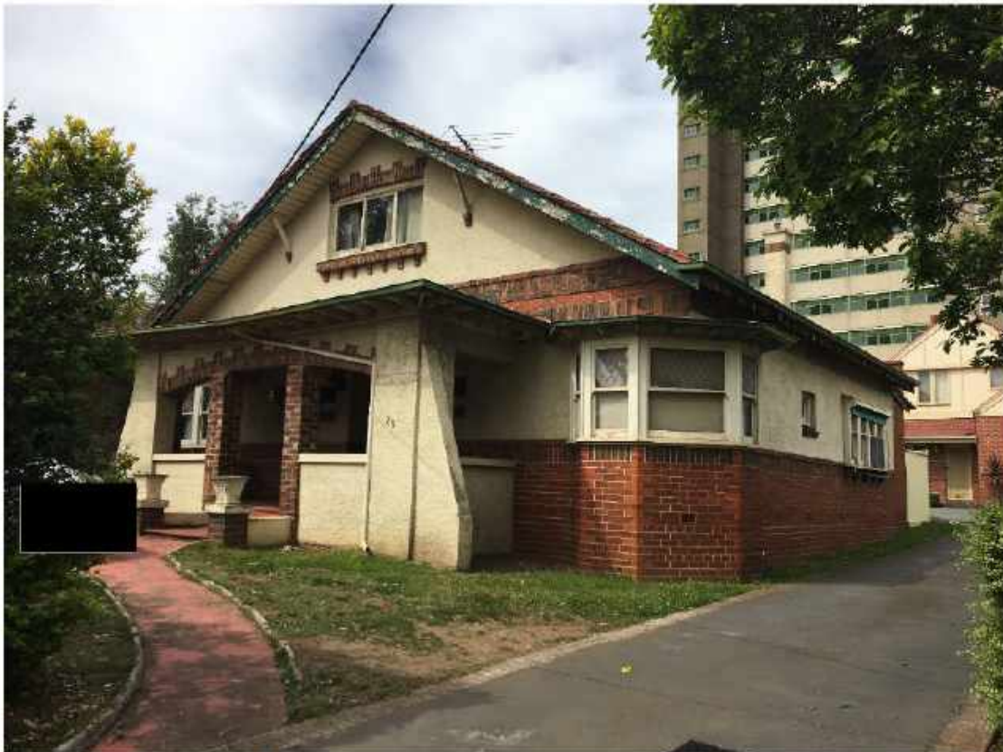
Figure 37. 20 Ascot Vale Road, Flemington, principal elevation (source: Context 2018)
