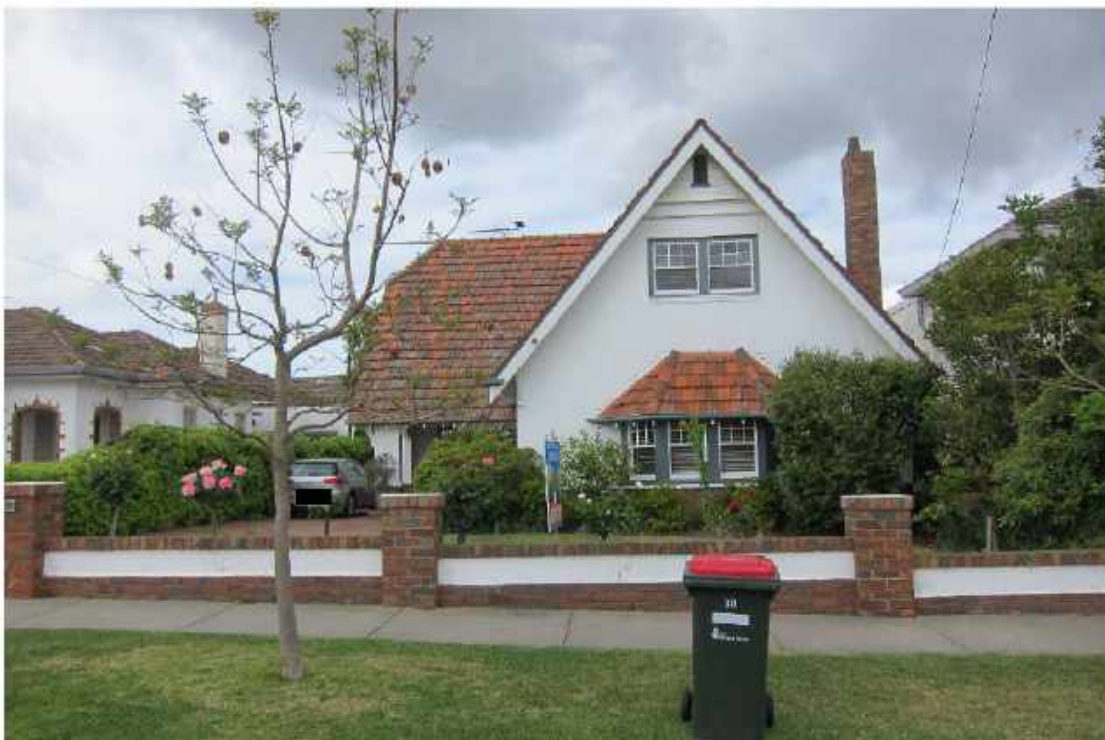
Figure 16. 30 Levien Street, Essendon, principal elevation (source: Context 2018)
