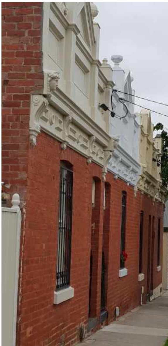
Figure 1. 1-7 Miller Street, Essendon, principal elevation
