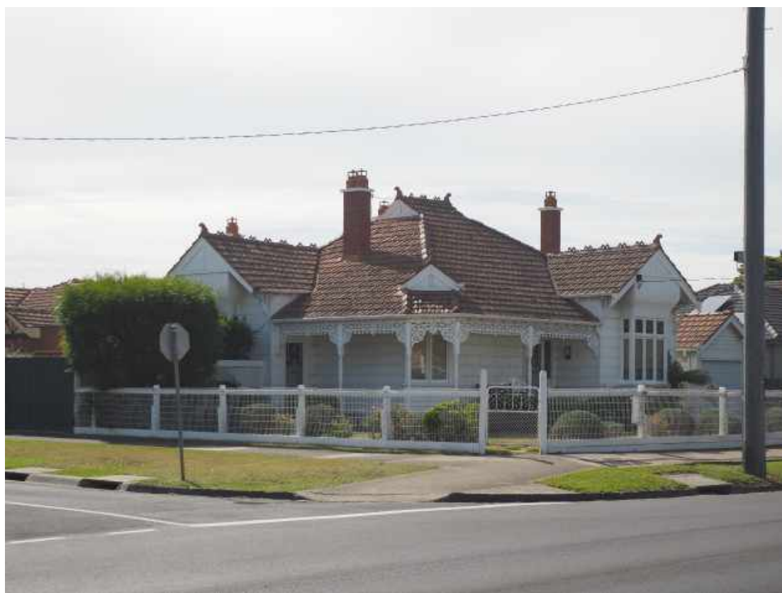
Figure 1. 330 Buckley Street, Essendon, south and west principal elevations (source: Context 2018)
