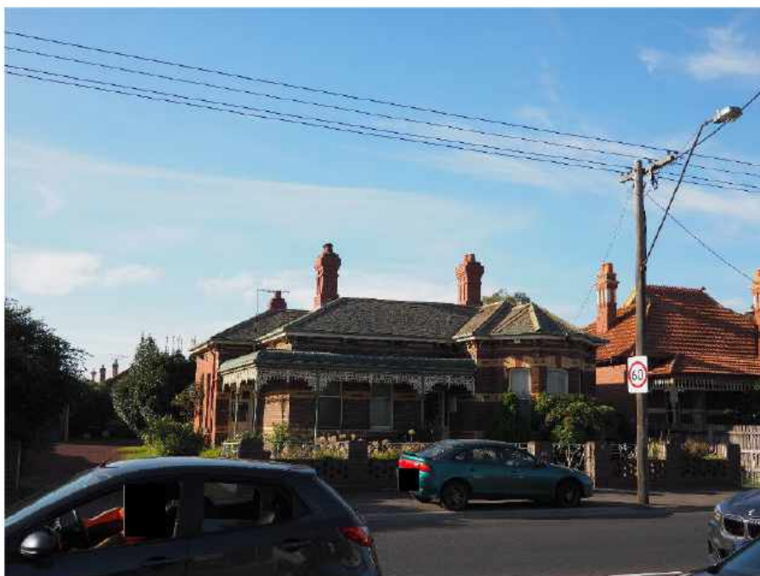
Figure 50. 40 Maribyrnong Road, Moonee Ponds, principal elevation (source: Context 2018)
