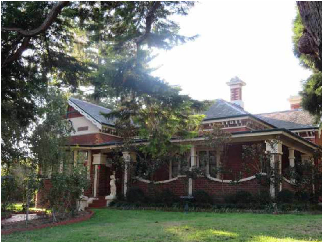
Figure 1. 57 Vanberg Road, Essendon, principal elevation (source: Context 2018)
