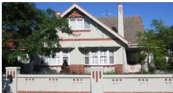
A highly picturesque and substantial Arts and Crafts bungalow with cross-ridged terracotta shingle -clad gable roof and attic storey windows in the gable ends.
