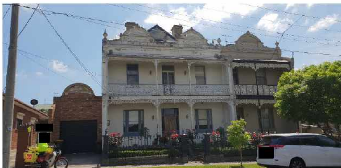
Figure 33. 14-16 Spencer Street, Essendon, principal elevation (source: Context 2018)
