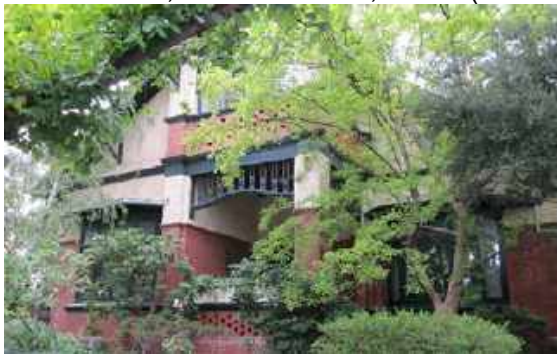
125 Wellington Street, Flemington, 1918 (HO126)
