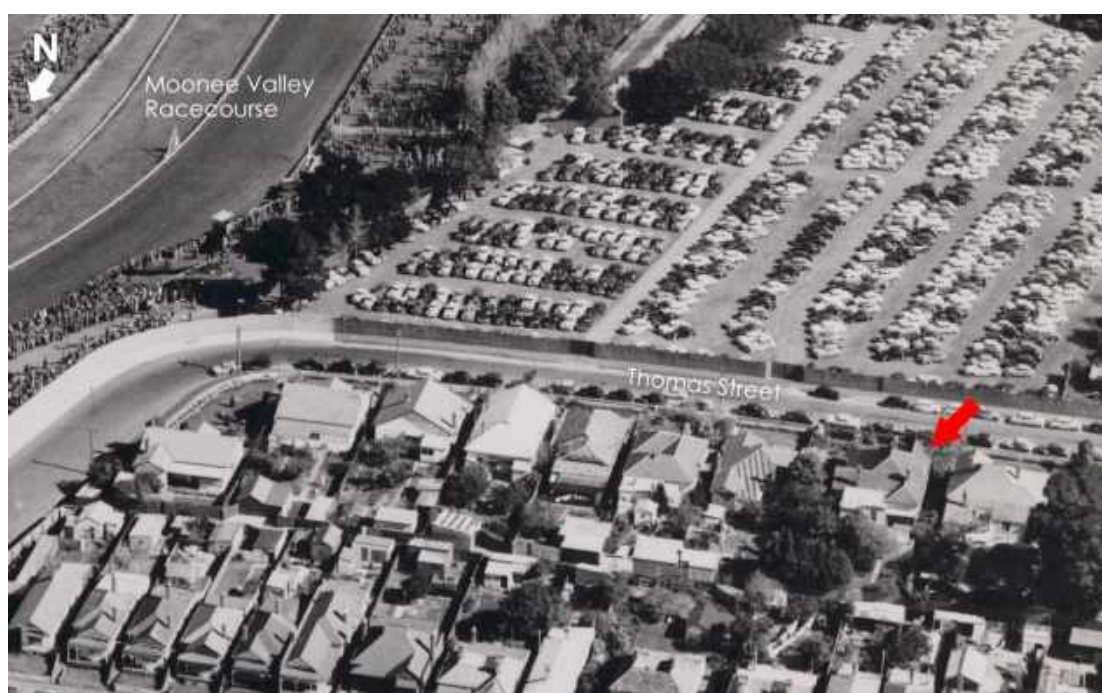
Figure 56. A section of an aerial photograph by Charles Pratt c1950s, showing 29 Thomas Street before the rear extension (source: State Library Victoria)
