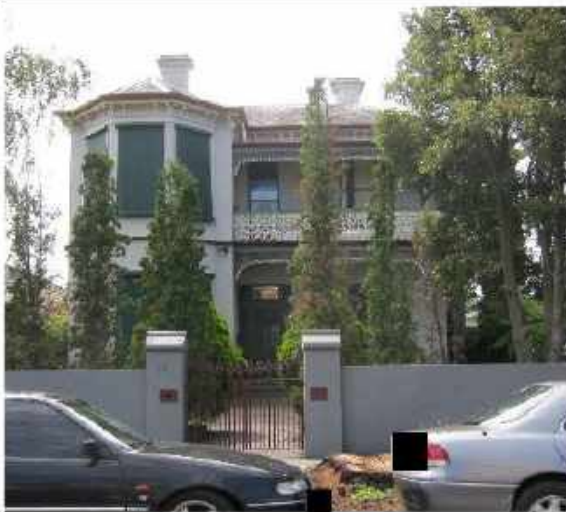
24 Grosvenor Street, Moonee Ponds, 1891 (HO230), is a representative two-storeyed asymmetrical Italianate villa with faceted bay to the projecting wing, bracketed eaves, hipped slate roof, chamfered reveals and two-storeyed cast iron lace corner verandah. The integrity of this place is high.
