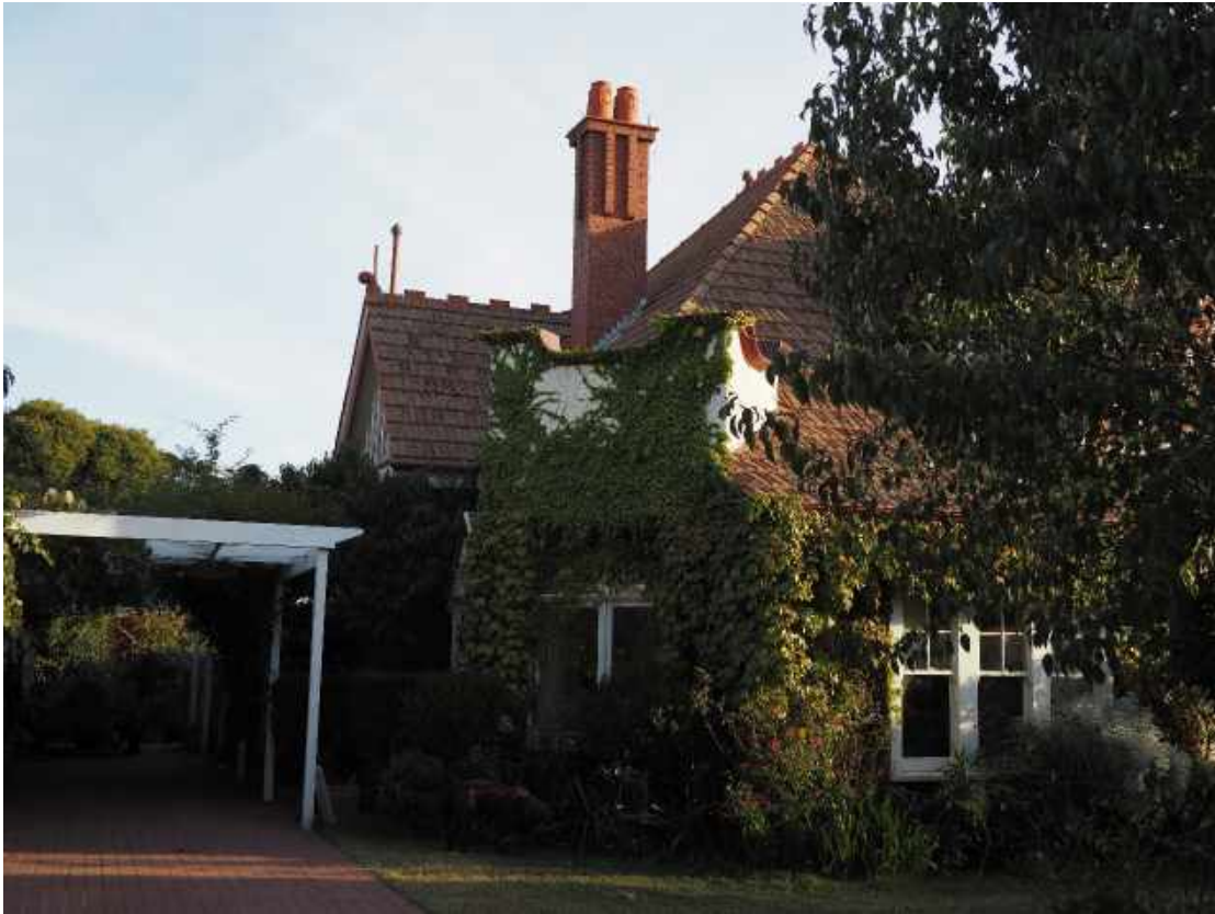
Figure 48. 83 Holmes Road, Moonee Ponds, north and east elevations (source: Realestate.com.au 2017)
