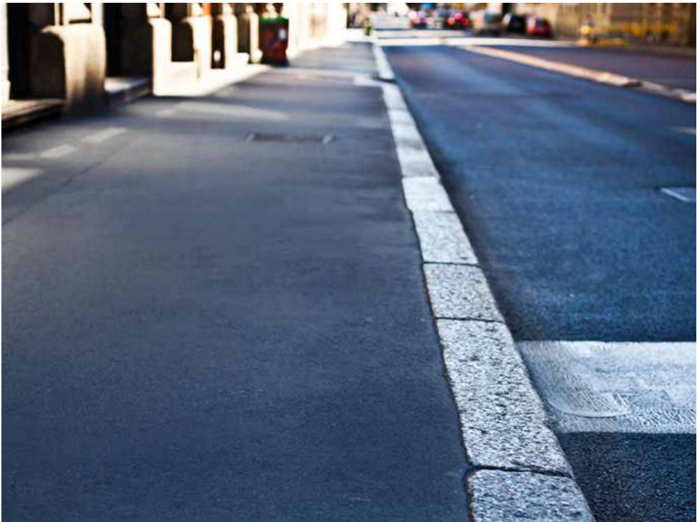
Example of asphalt footpath
