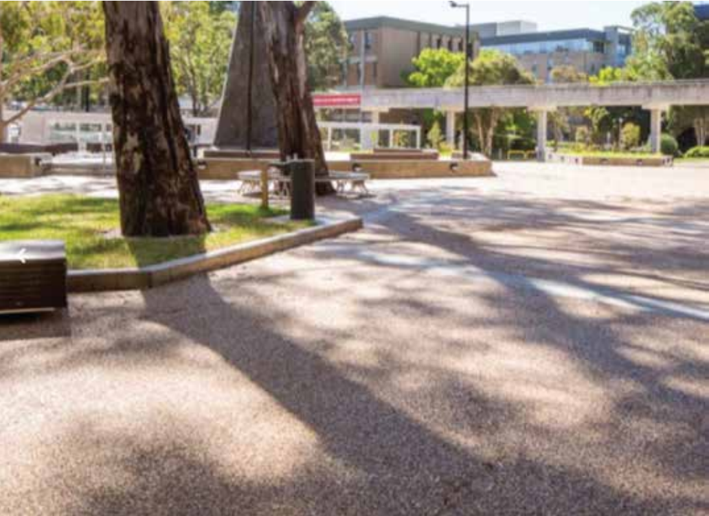
Example of porous paving
